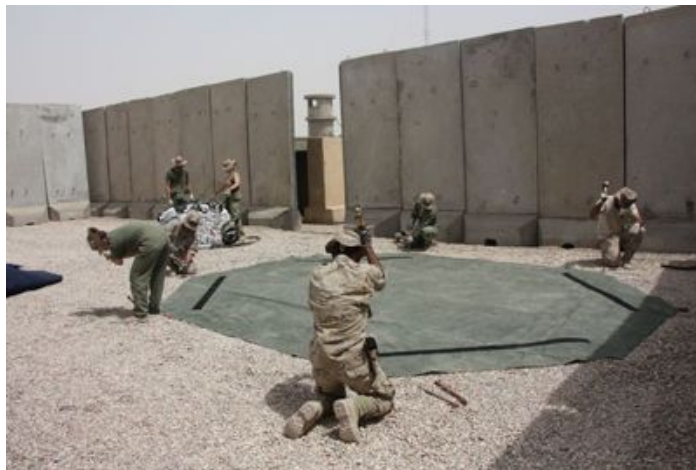
FIG. 6 Construction of the war theatre military FOB between FP T-Walls
